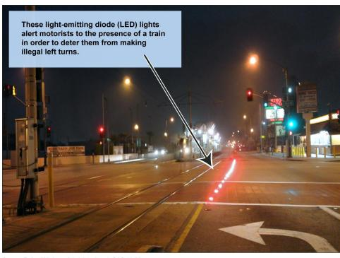
Figure 4: Photos of In-Roadway Lights That Delineate a Grade Crossing
